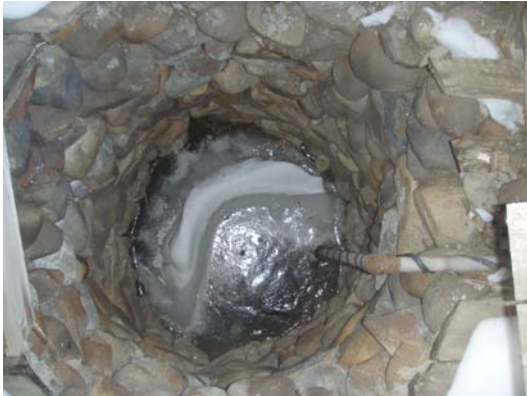
Hand dug well, 5' to water surface, Building F-1
