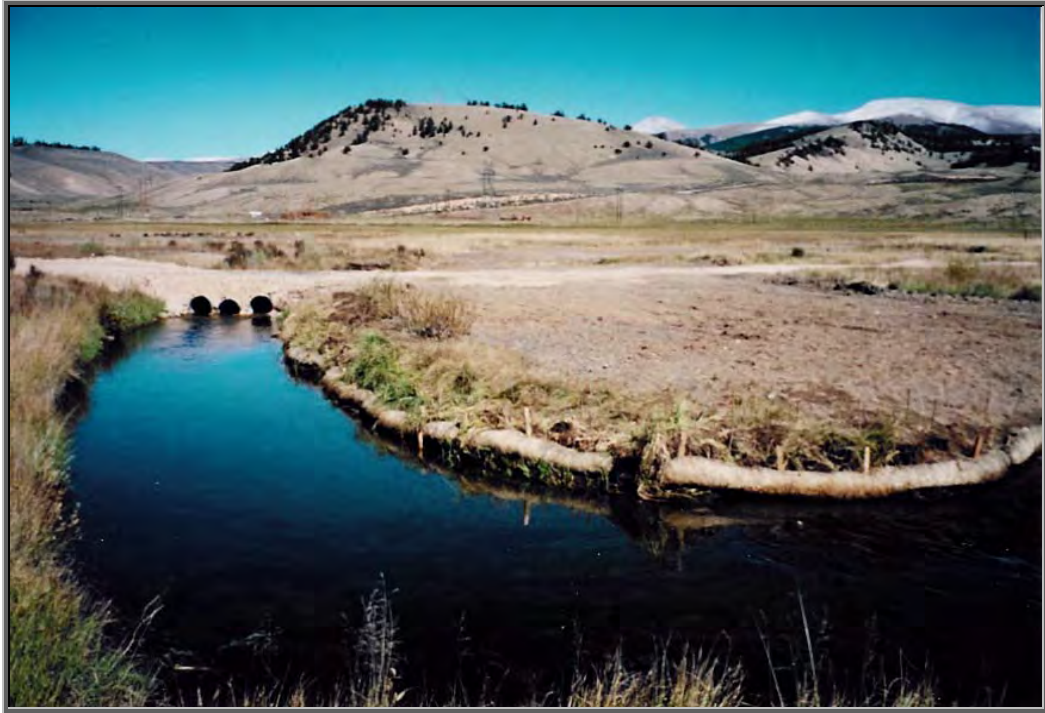
Soil amendment, bank stabilization, and revegetation.
