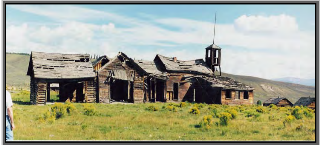
r "Vigilante" Tower of the Derry Homestead
